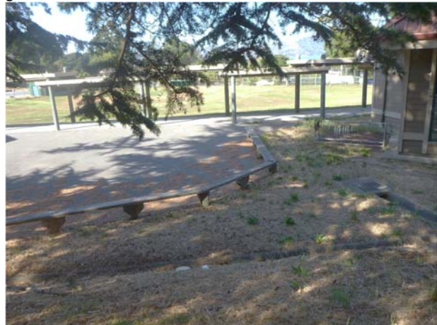
Figure 7. Photo looking downstream at downstream extent of Phase 1A.
