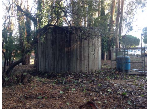
Figure 5. Existing water tank infrastructure in eucalyptus grove.
