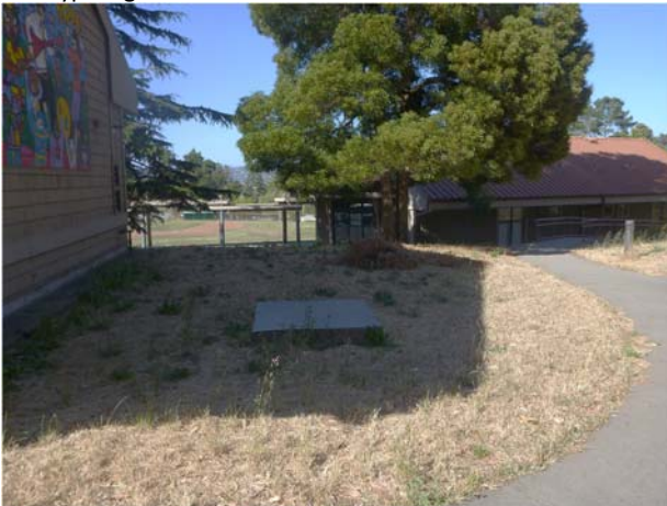
Figure 6. Photo looking downstream at path between school buildings.
