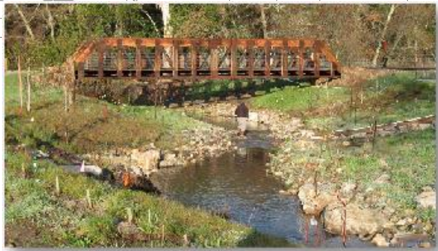
TIMBER BRIDGE STREAM CROSSING
