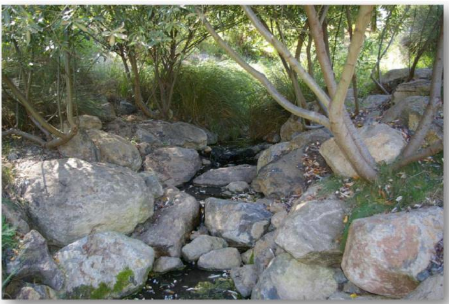
BOULDER CHUTE WITH WILLOW PLANTINGS
